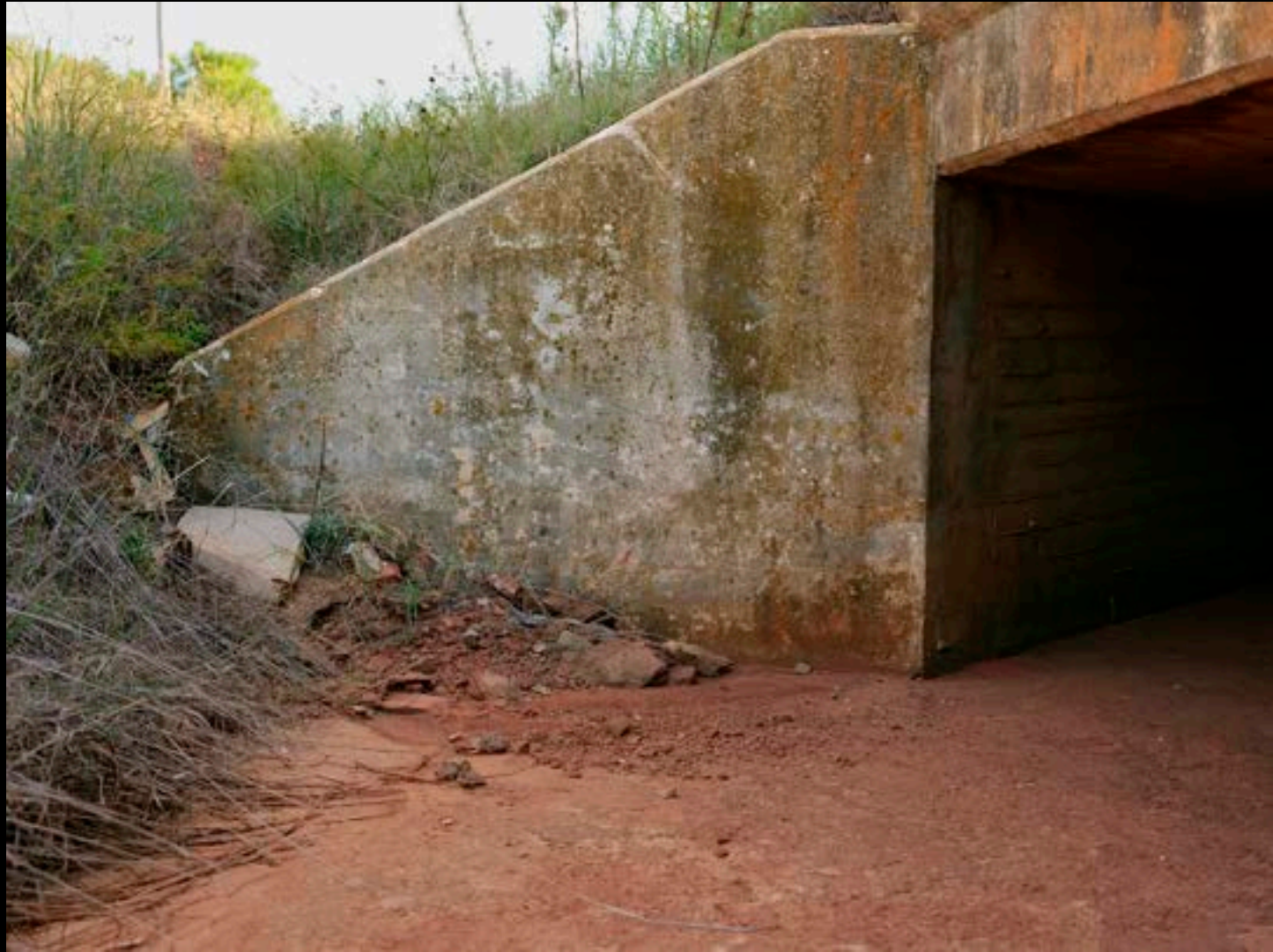
Culvert where Karen Silkwood died
