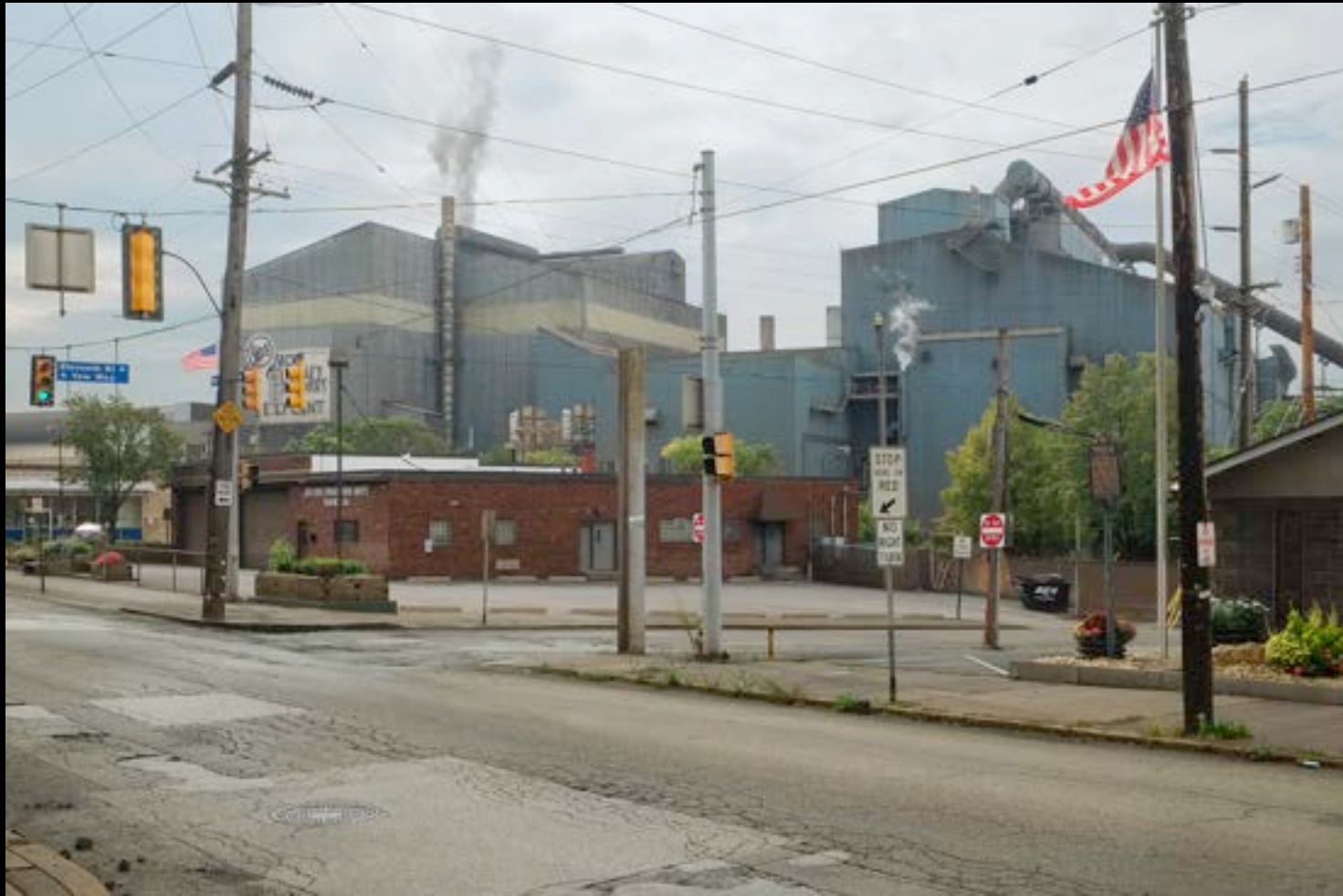
Braddock, PA steel plant that took part in the strike
